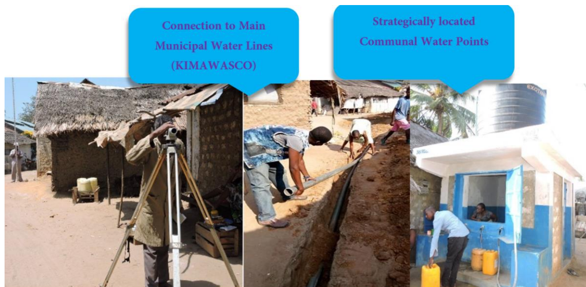
Figure 20: Connection of the water kiosks to the water lines
